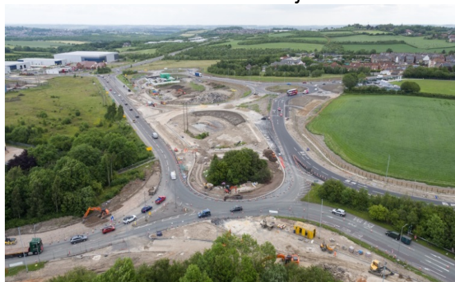
Northwards view of work at new junctions
